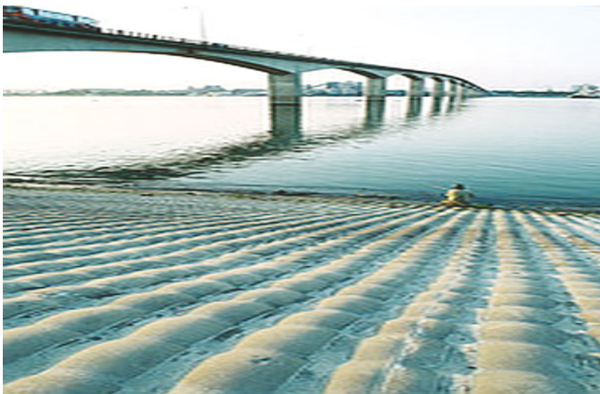
Fig 14.1 Geo-textile bags with Cement at the banks of Meghna River at Meghna Gumti Bridge
