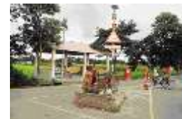
Figure 4: Intersection was treated by putting an island and installing signage with chevron marking
