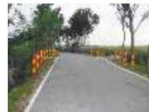
Figure 10: Newly constructed culverts
