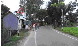
Figure 13: Appropriate signage and markings were put
