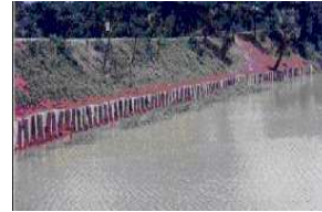
Figure 2: Adequate protective work was undertaken
