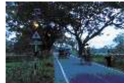
Figure 8: Proper grade & adequate signage were placed
