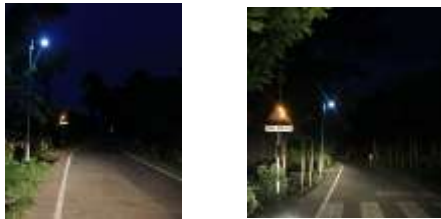
Figure 22: Solar signage and Street lights along with edge marking
