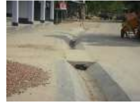
Figure 6: Constructed V-shaped drains
