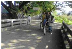
Figure 7: Grades of the approach were not suitable for NMTs
