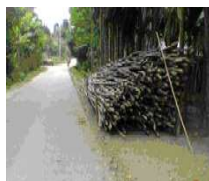
Figure 17: Shoulder encroached with hazardous materials
