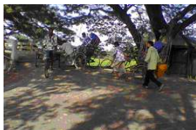
Figure 3: Improper Grade and Interfacing, intersection vision obscured by the big tree and the structure, no signs
