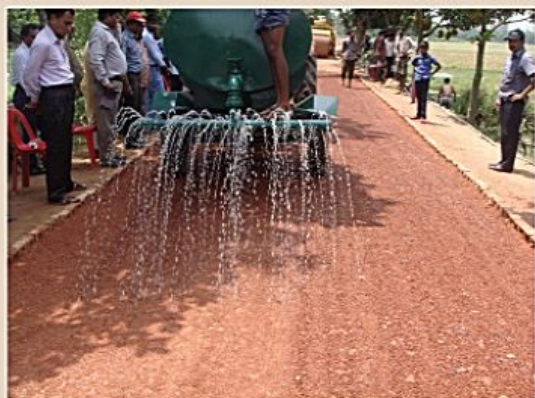
Practical demonstration of OJT on base course construction at Naogaon by CQCL Engineers
