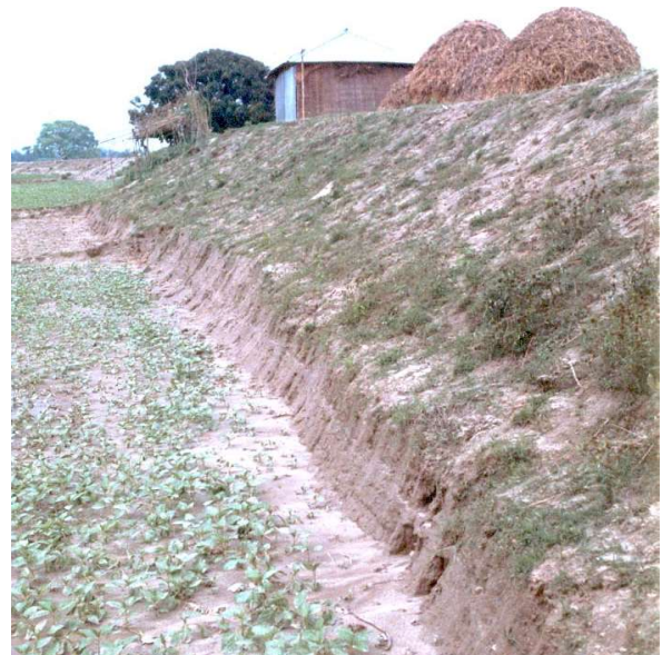
Figure-22 Cutting of Toe of Embankment
