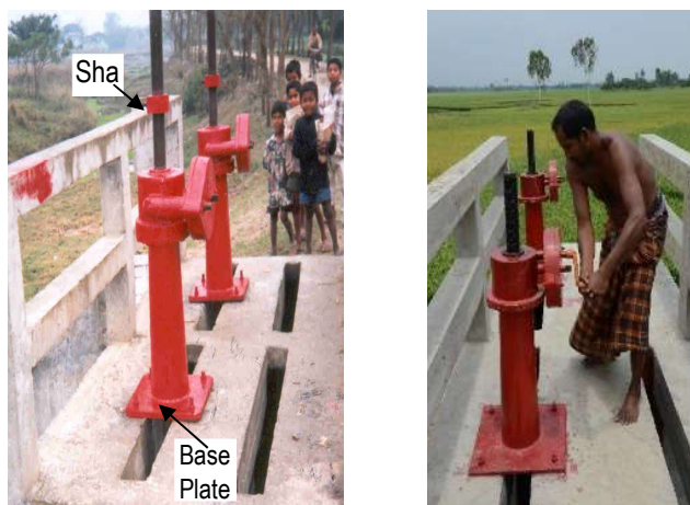
Figure-13 Raising of Vertical Gate
