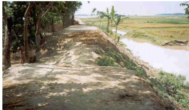
Figure-20 Settlement of Crest and side slope
