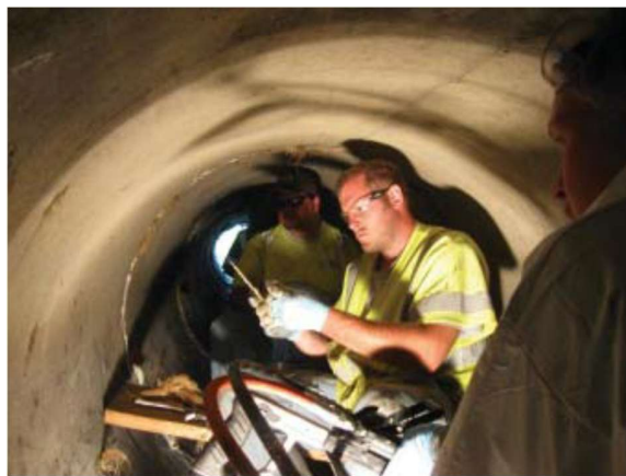
Sealing a pipe joint from the inside with activated oakum (jute fibers soaked with a resin)
