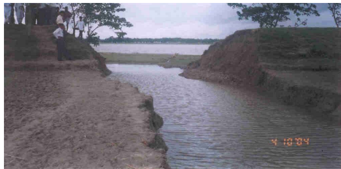
Figure-33 Embankment Breaching
