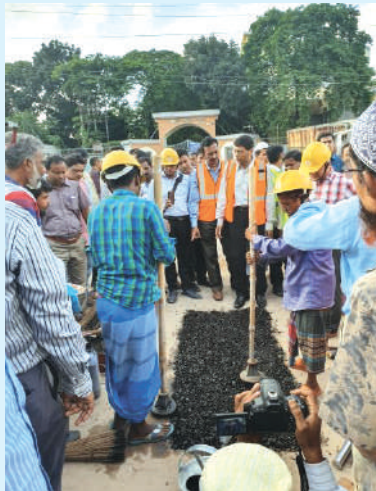
Demonstration of "On-the-Job training on road surface repair using bituminous material" is going on in presence of Mr. Nur Hossain Hawlader, SE, Dhaka Region and Executive Engineer, Dhaka district.
