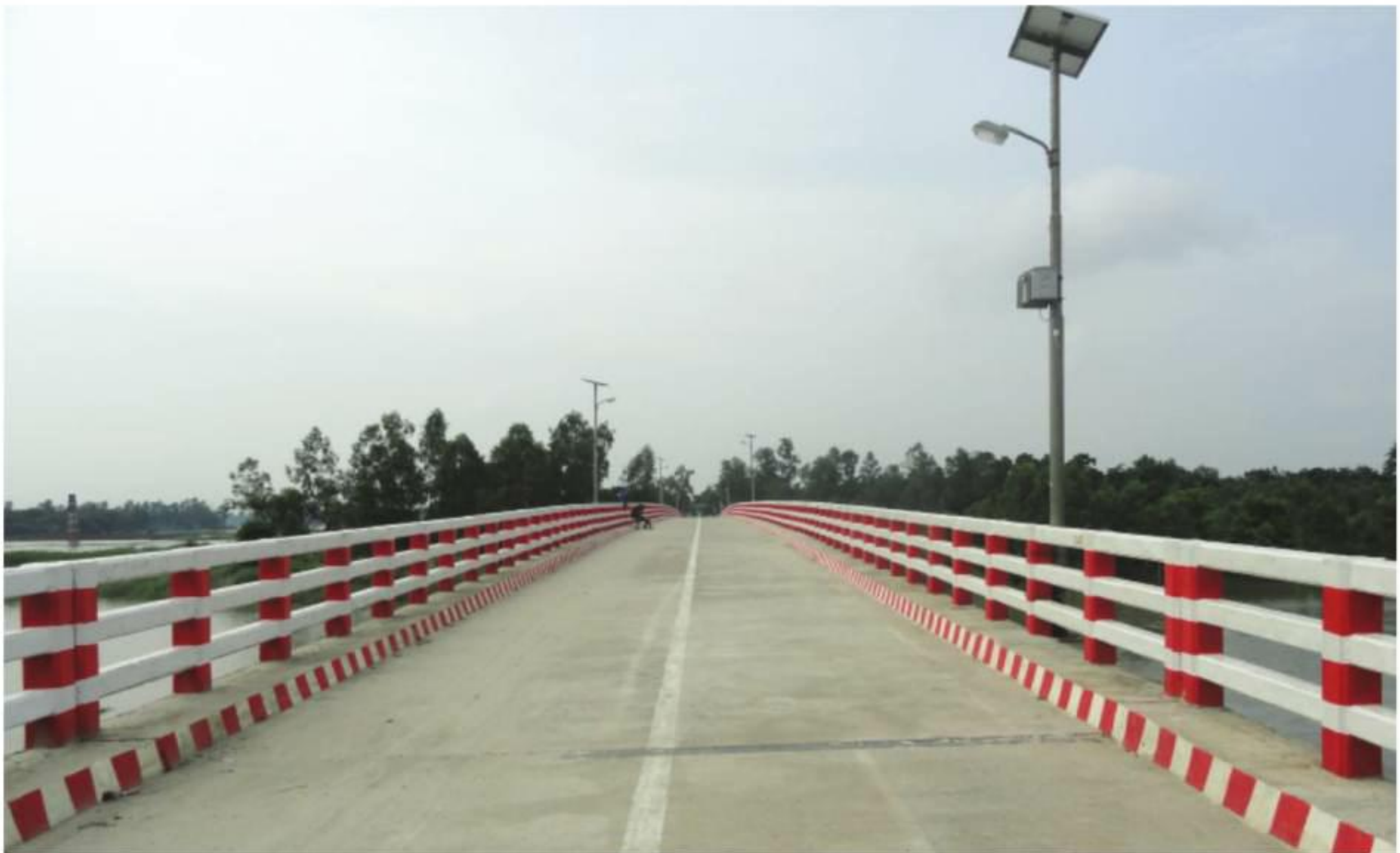
300 meter long PC girder bridge on Bangshai river on Mirzapur-Patharghata road under Mirzapur upazila in Tangail district.
