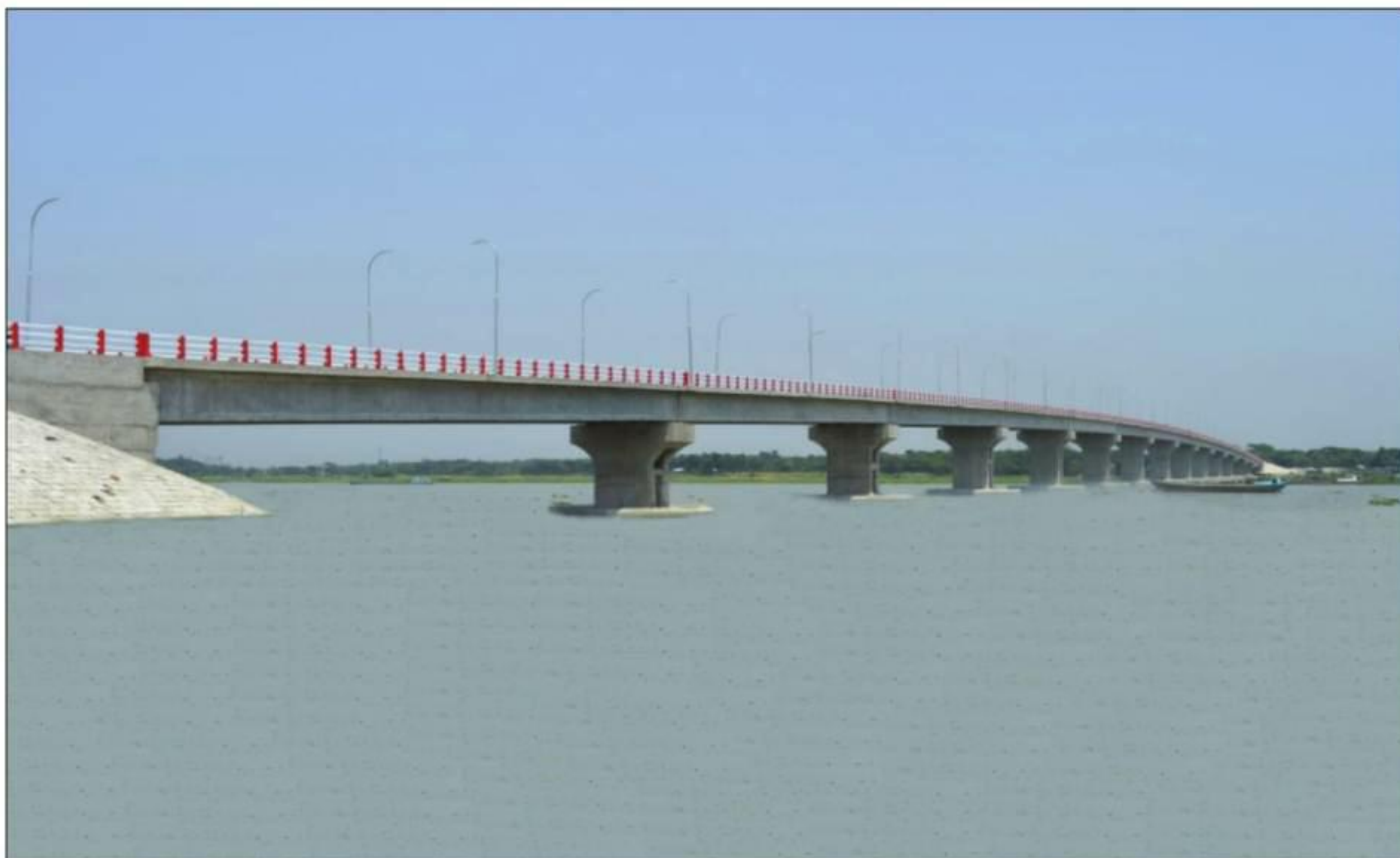
588.65 meter long pre-stressed concrete girder bridge on Modhumoti river at Chapail ghat on Gopalganj-Singati road under Gopalganj sadar upazila
