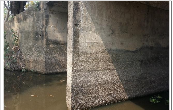
Wing Wall treated as Sub-Structure Component
