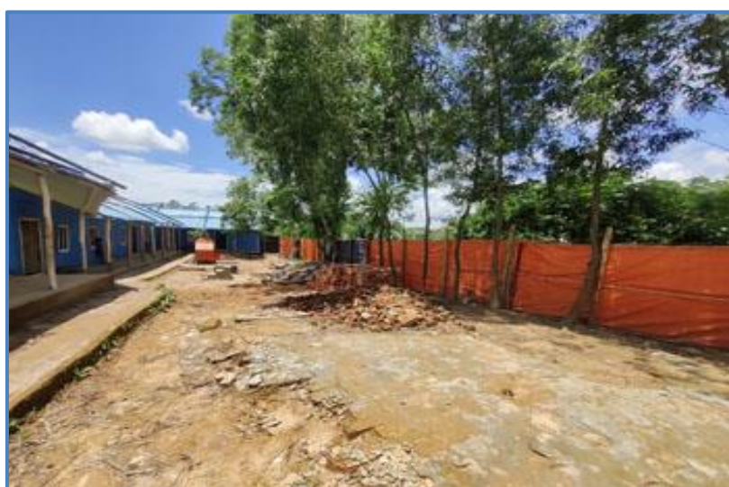
Figure 1.5.2: Proposed location of Satellite Fire station construction
