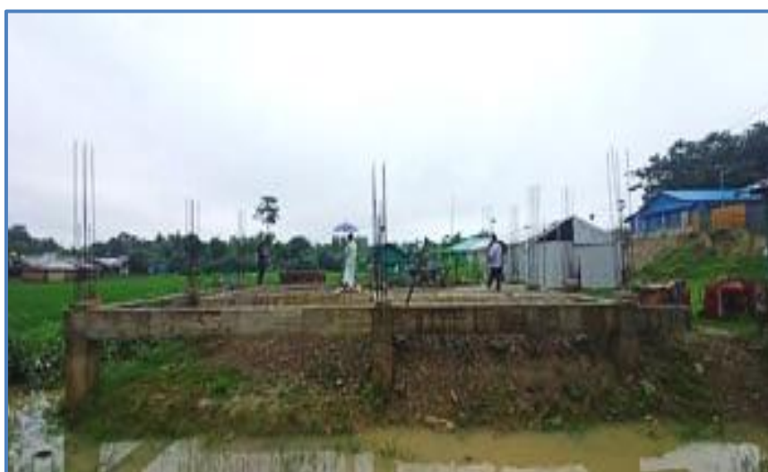
Figure 1.5.2: Proposed location of Fire service station construction
