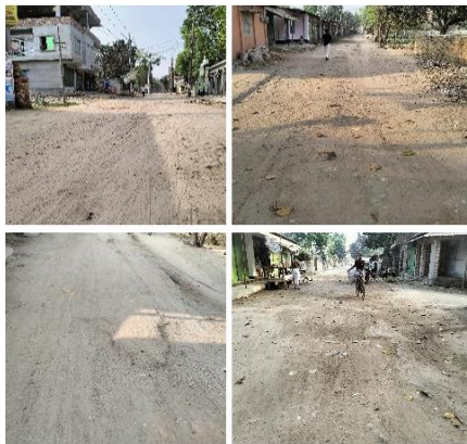
Existing Road Condition of the Subproject Site
