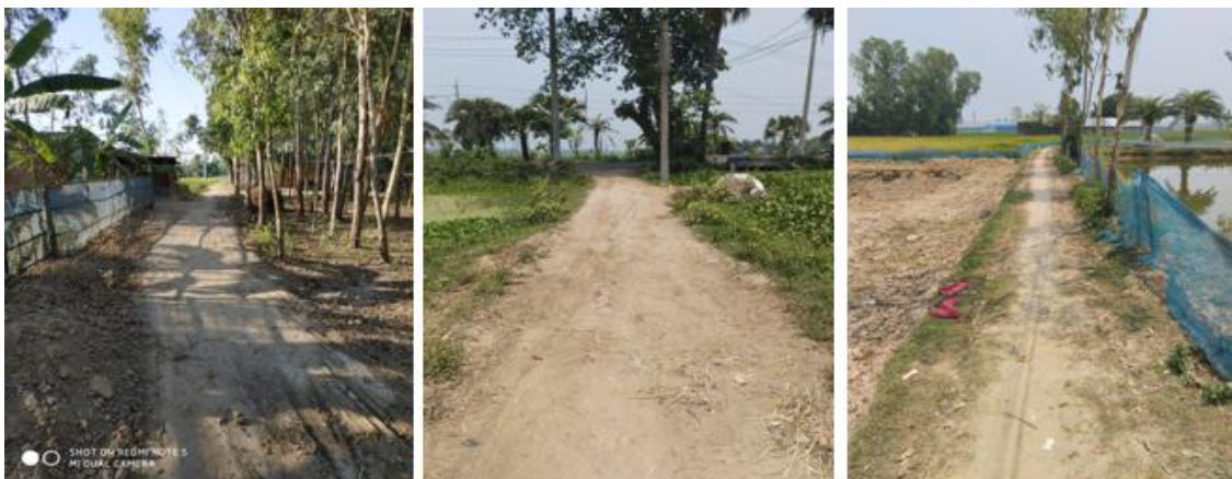
Existing Road Condition of the Subproject Site
