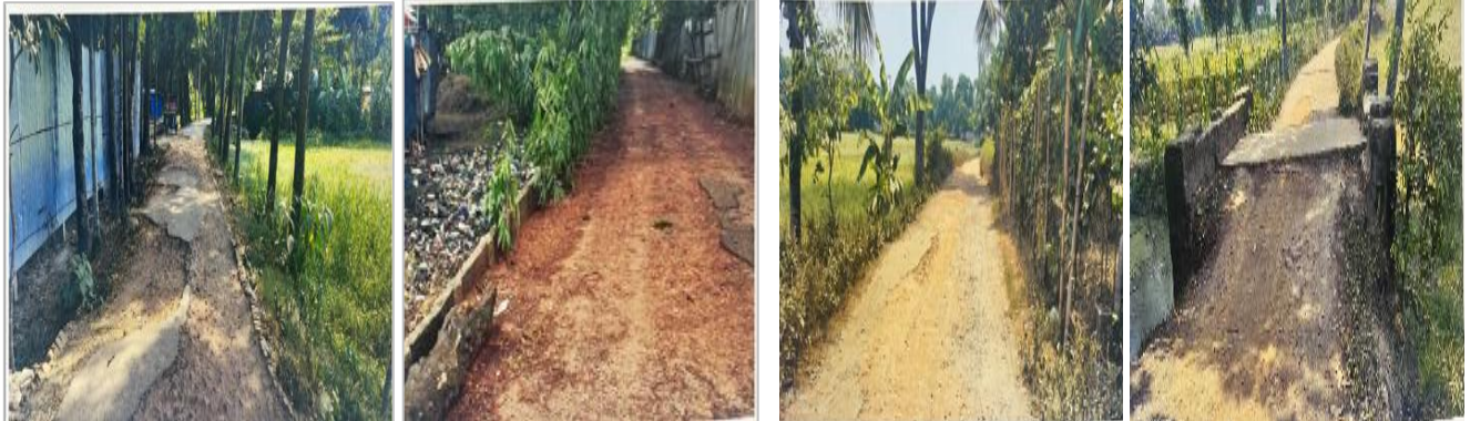
Existing Road Condition
