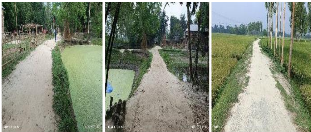
Existing Road Condition of the Subproject Site
