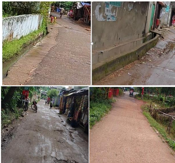
Existing Road Condition with Drain
