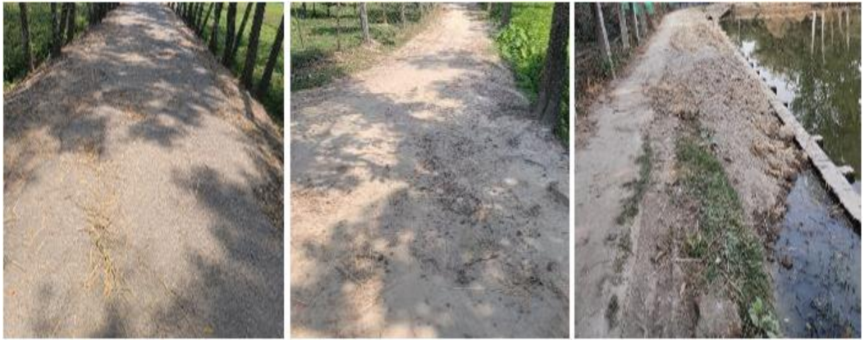
Photographs 3.1: Existing Road Condition of the Subproject Site
