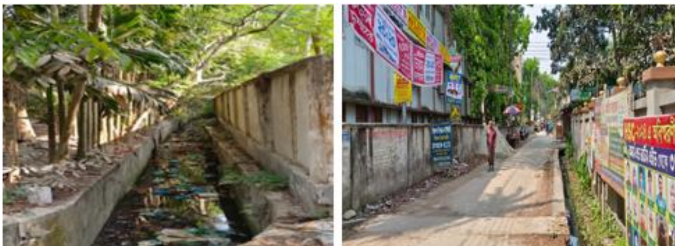
Photographs: Existing Drain Condition of the Subproject Site
