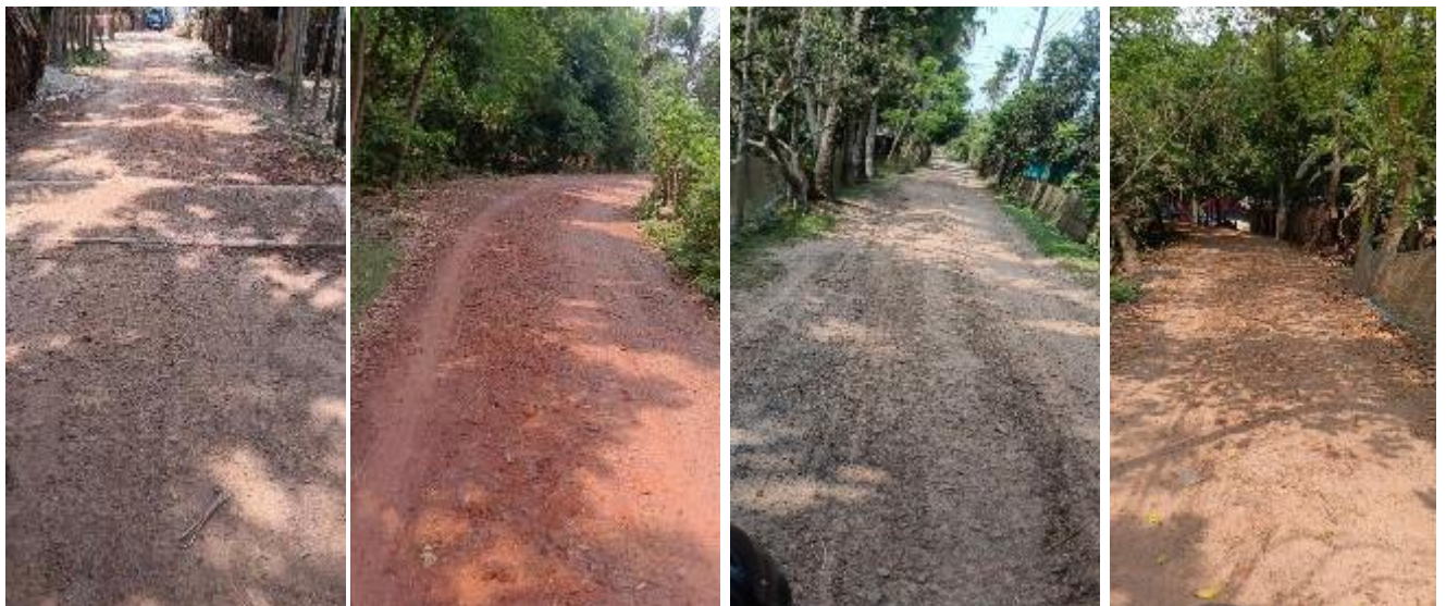
Photographs: Existing Road Condition of the Subproject Site
