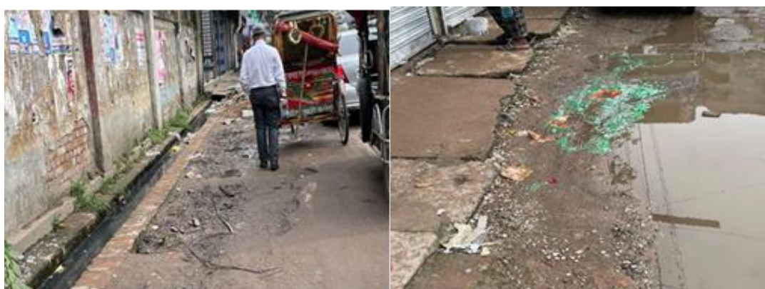
Photograph 2.2.2: Existing Drain Condition of the Subproject Site
