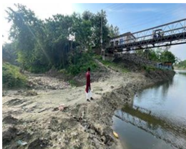
Photograph 2.2.3: Existing Outfall Condition of the Subproject Site
