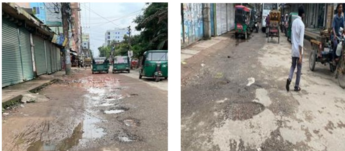
Photograph 2.2.1: Existing Road Condition of the Subproject Site
