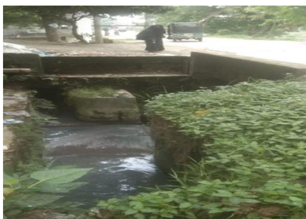
Photograph 2.2.3: Existing Outfall Condition of the Subproject Site
