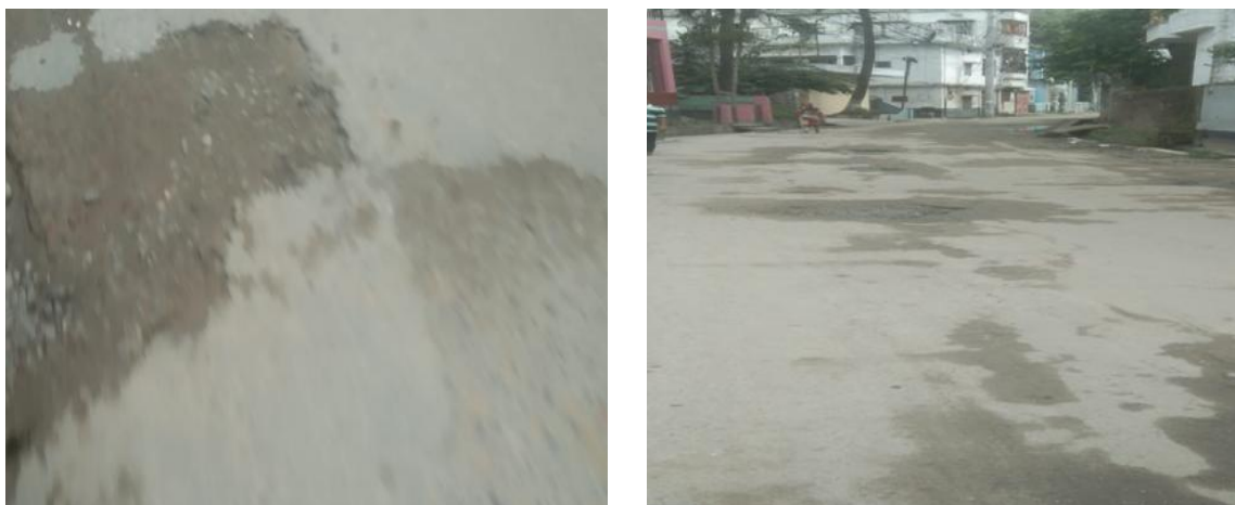
Photograph 2.2.1: Existing Road Condition of the Subproject Site
