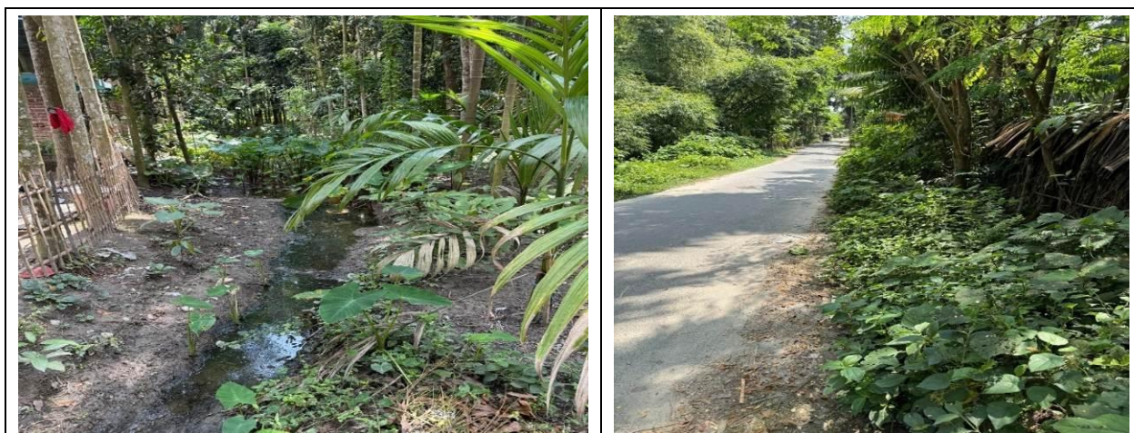
Photograph 2.2.2: Existing drain Condition of the Subproject Site
