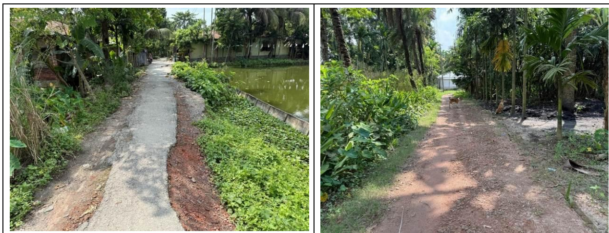
Photograph 2.2.1: Existing Road Condition of the Subproject Site
