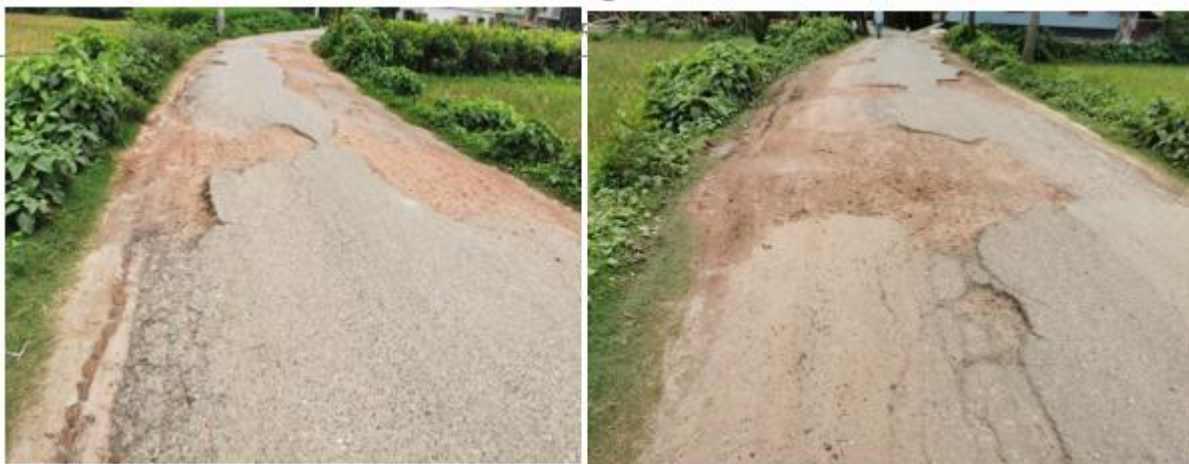
Photograph 2.2.1: Existing Road Condition from Gulshanmore to Jamalgonj road via Teghar Railgate of the Subproject Site
