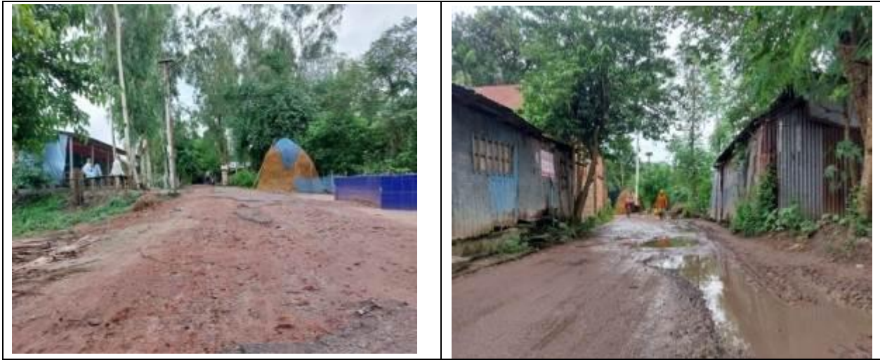
Photograph 2.2.1: Existing Road Condition of the Subproject Site
