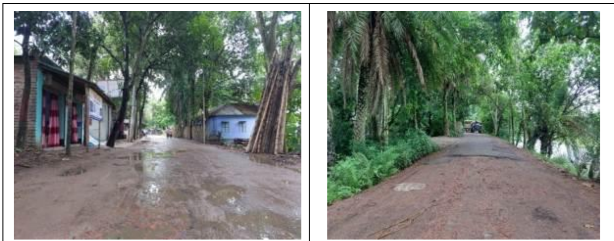
Photograph 2.2.3: Existing Outfall Condition of the Subproject Site
