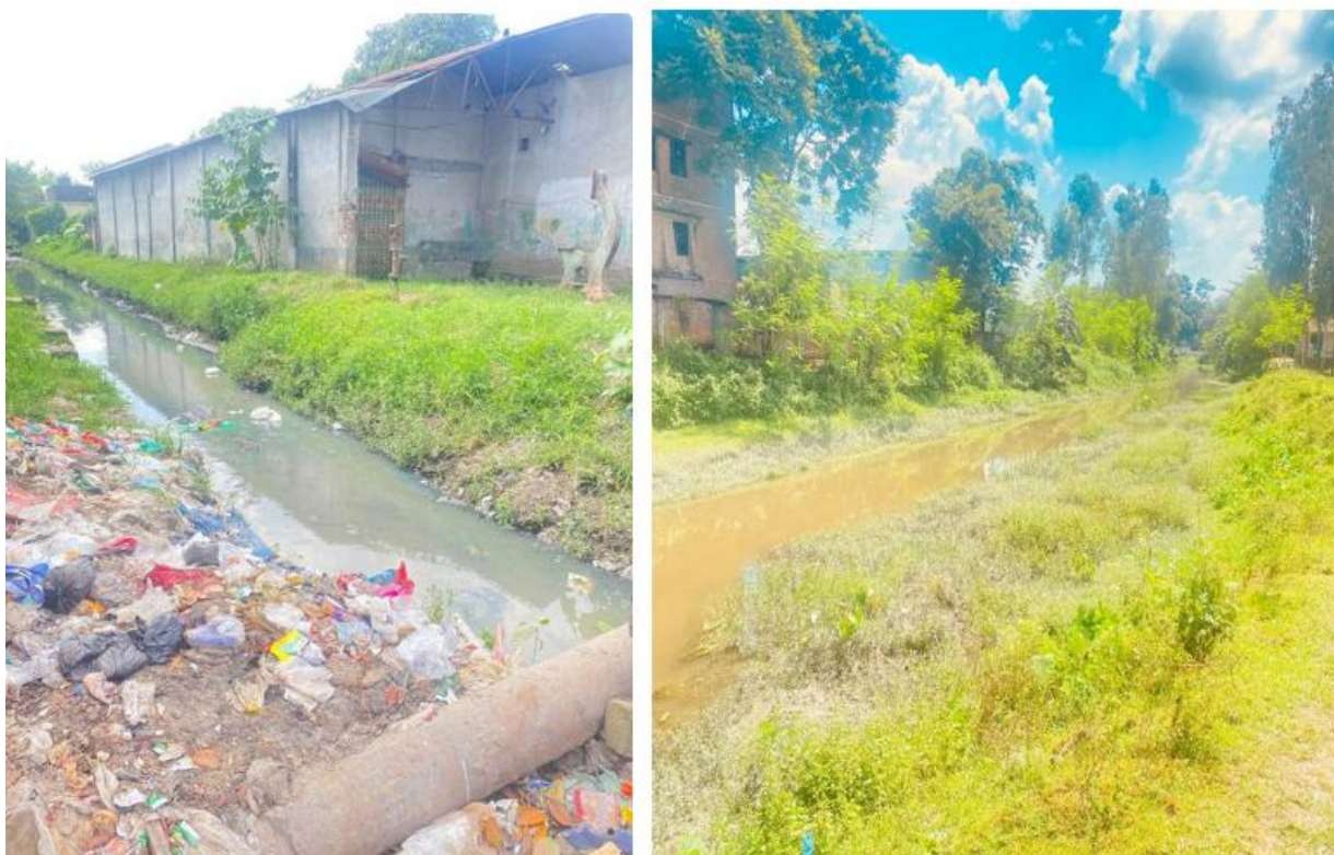
Photograph 2.2.3: Existing Outfall Condition of the Subproject Site
