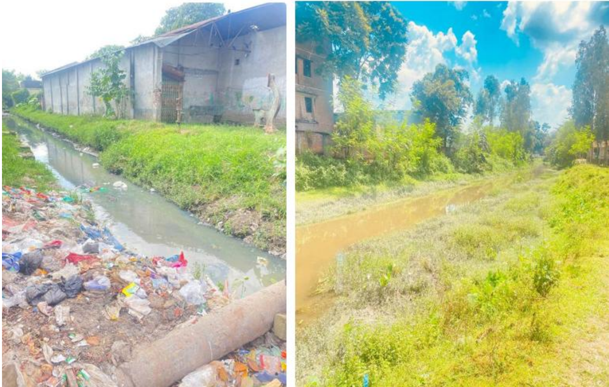
Photograph 2.2.3: Existing Outfall Condition of the Subproject Site
