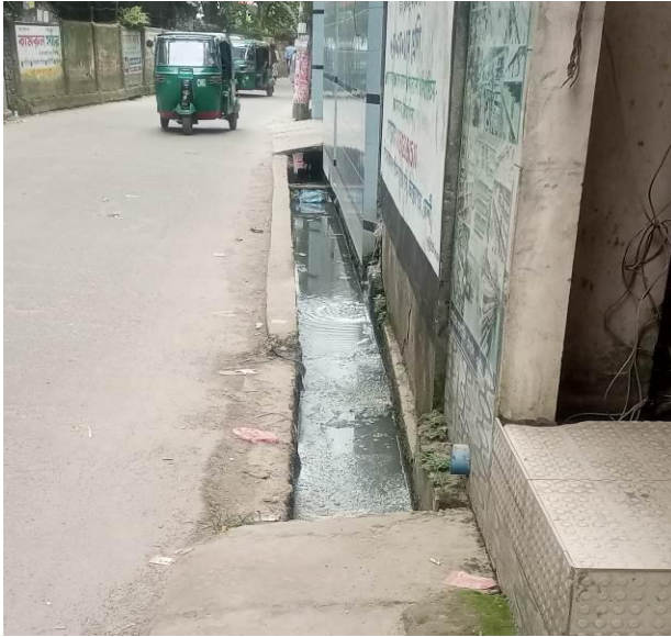
Photographs 2.2.1(b): Existing Drain Condition at Doctorpara Road of the Subproject Site
