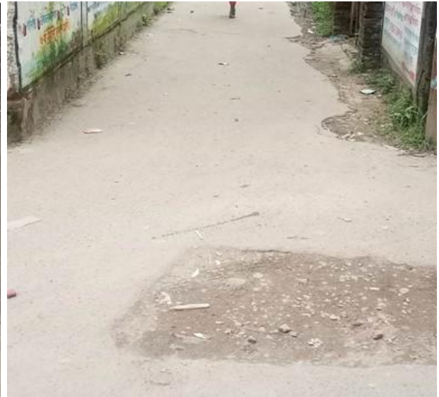
Photographs 2.2.1(h): Existing Road Condition at District Arts Academy Road
