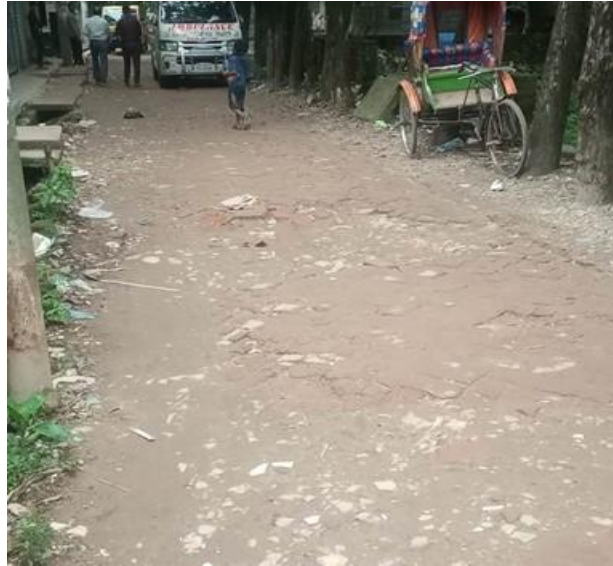
Photographs 2.2.1(j): Existing Road Condition at Pathan Bari Road of the Subproject Site
