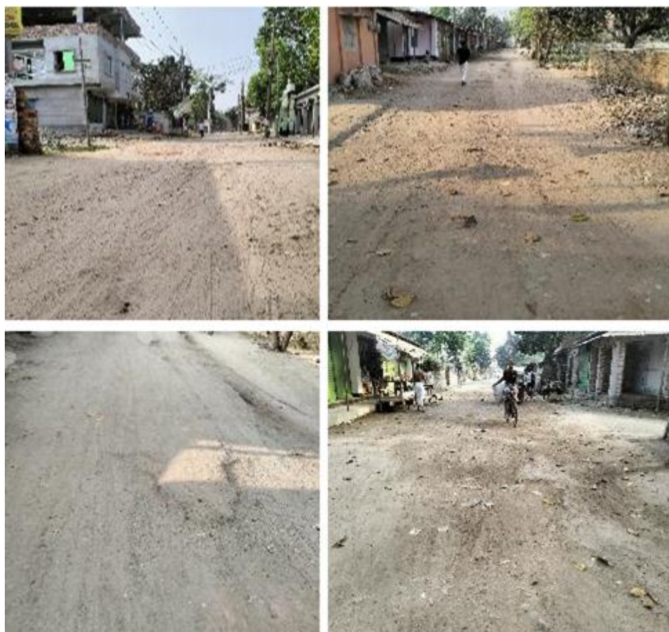
Photograph 2.2.1: Existing Road Condition of the Subproject Site
