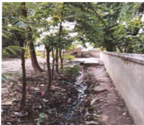
Photograph 2.2.2: Existing Drain Condition of the Subproject Site
