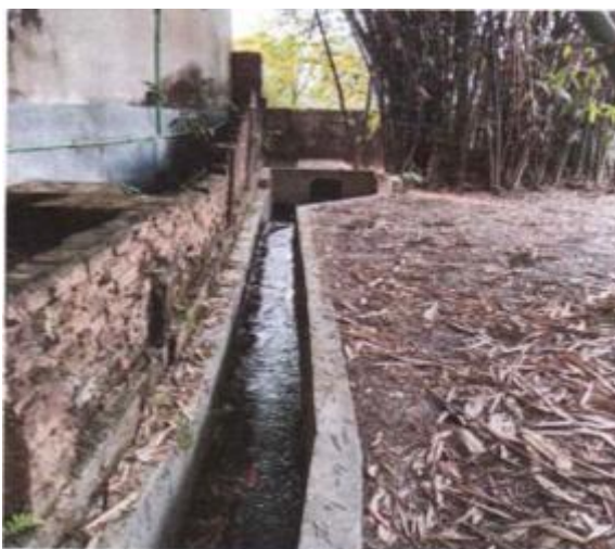
Photograph 2.2.3: Existing Outfall Condition of the Subproject Site
