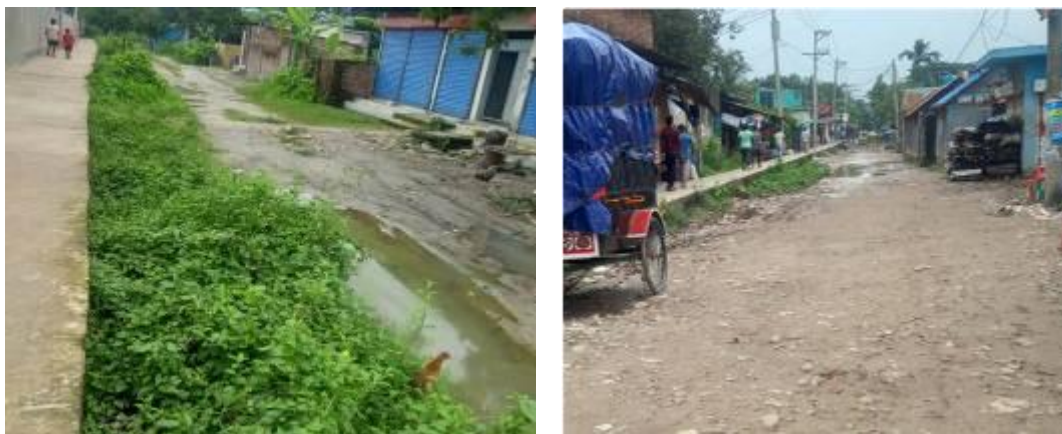
Photograph 2.2.1: Existing Road Condition of the Subproject Site
