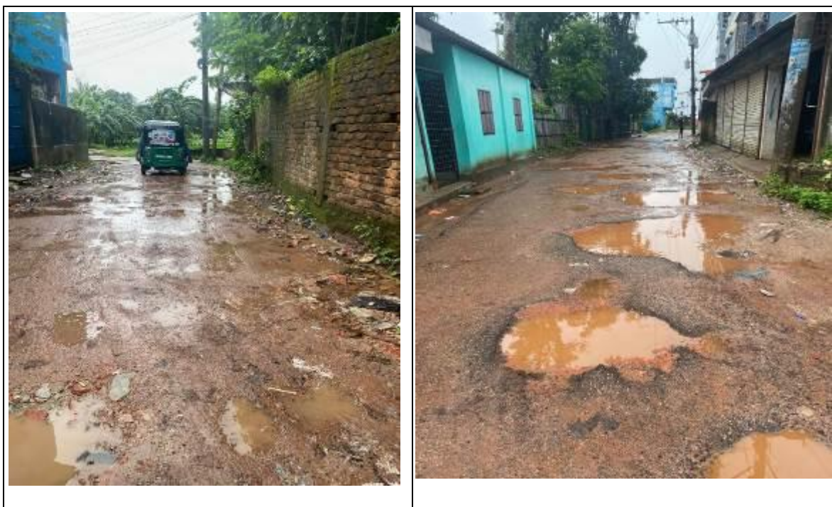
Photograph 2.2.1: Existing Road Condition of the Subproject Site
