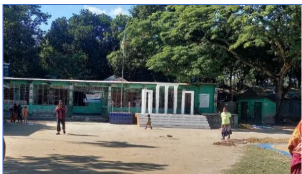
Figure 6: Existing school Building
