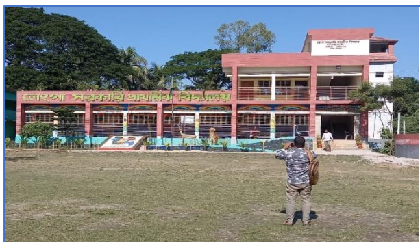
Figure 6: Existing school Building
