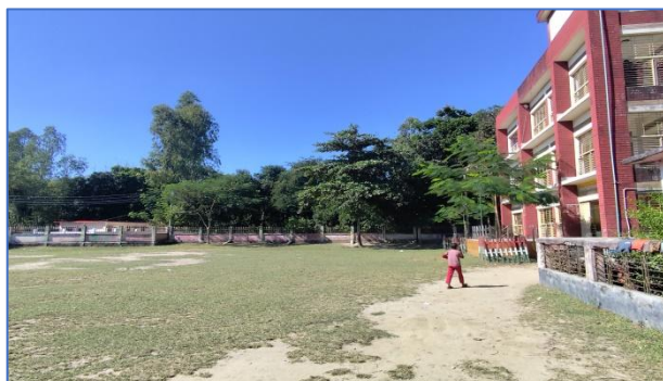
Figure 3: Current Situation of the Existing Subproject Site
