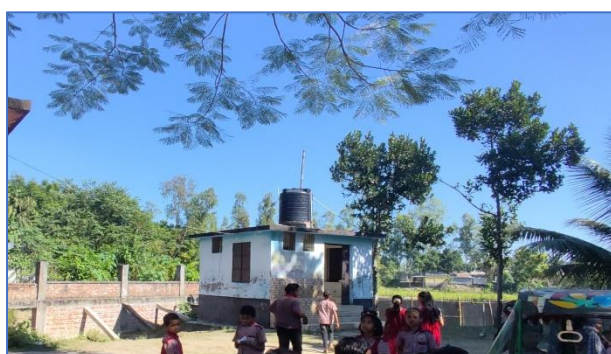
Figure 7: Wash Block need to be Demolish
