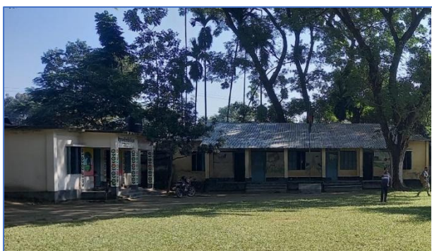
Figure 6: Existing school Building
