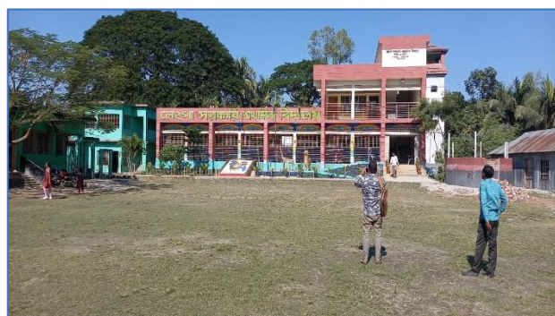
Figure 3: Current Situation of the Existing Subproject Site
