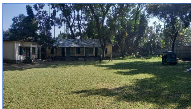
Figure 3: Current Situation of the Existing Subproject Site
