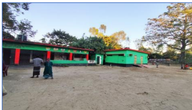
Figure 3: Current Situation of the Existing Subproject Site
