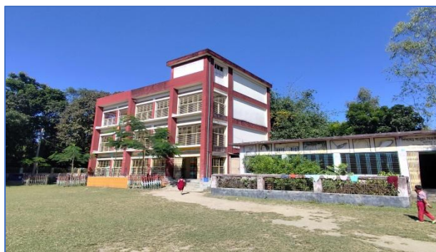
Figure 6: Existing School Building
