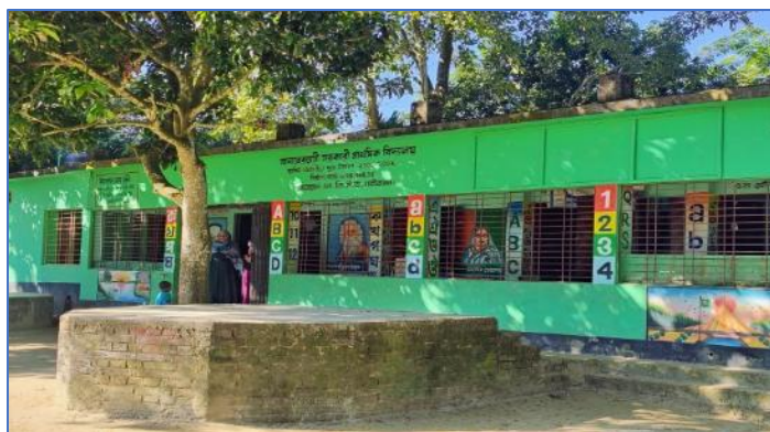
Figure 7: Existing School Building
