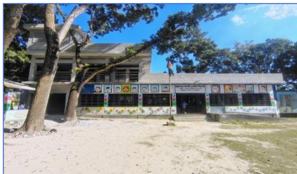
Figure 6: Existing School Building
