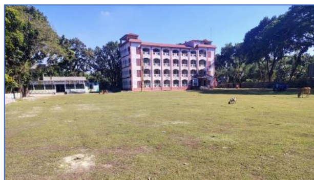
Figure 3: Current Situation of the Existing Subproject Site
