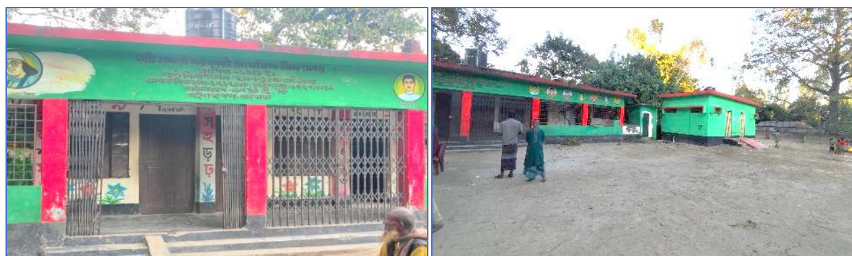
Figure 7: Existing School Building
