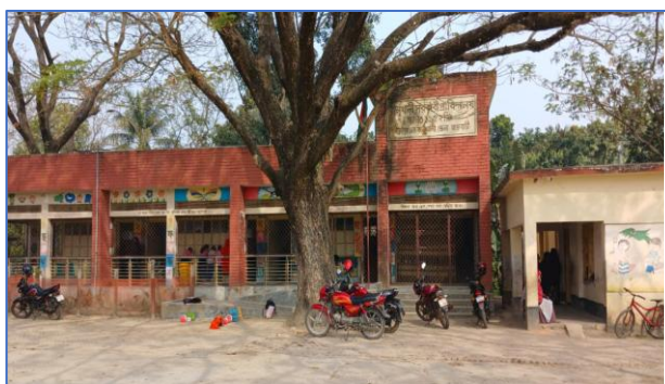
Figure 6: Existing School Building
