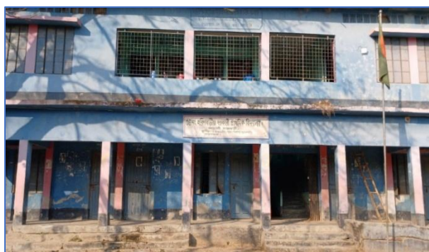
Figure 7: Existing School Building
