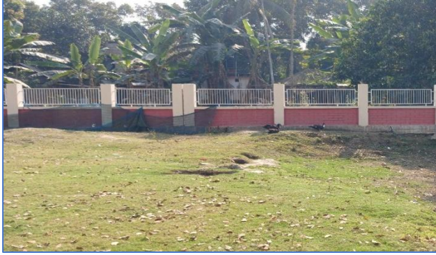
Figure 5: Proposed Material Storage Area
