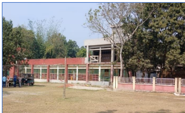
Figure 7: Existing School Building
