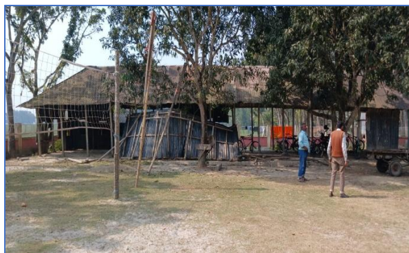
Figure 8: Tin-Shed School required Demolition
