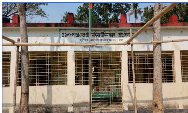
Figure 7: Existing School Building
