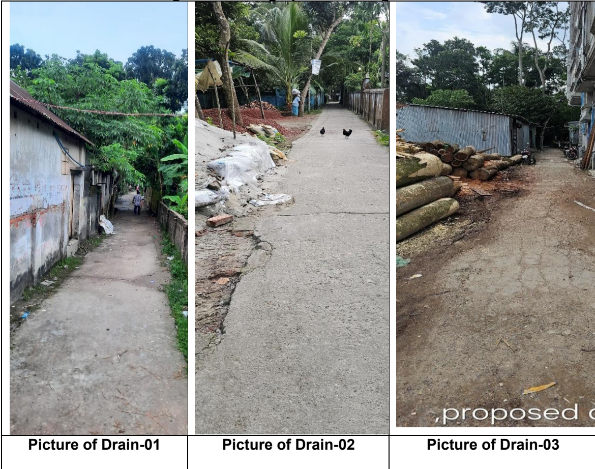
Figure 5: Photograph of Existing Drains
