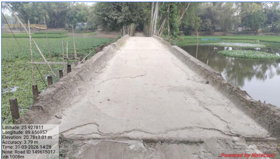
Starting Point of Khamar Hasnabad School-Burirhat Road
