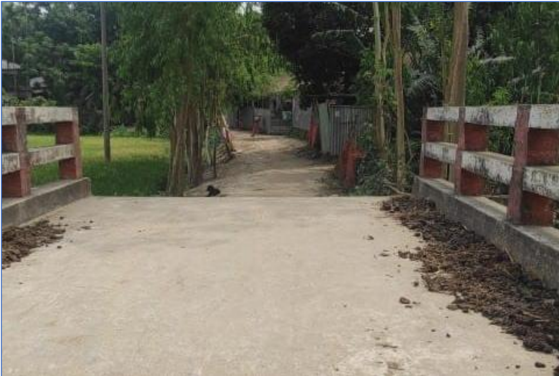
Starting Point of New Jorgach - BWDB Embankment at kharkharia Road
