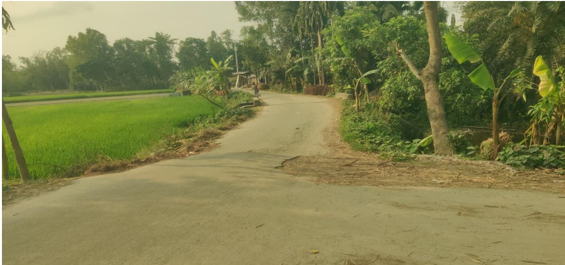
Starting Point of Hindupara to Hamurhat Road
