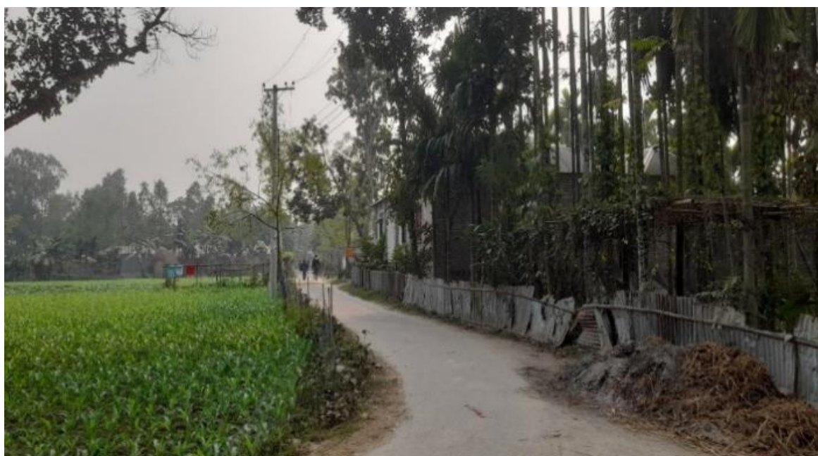
Starting Point of Improvement of Bhangamore GPS Flood Shelter Community Road from Chander Bazar-Rasulpur-2 GPS Road
