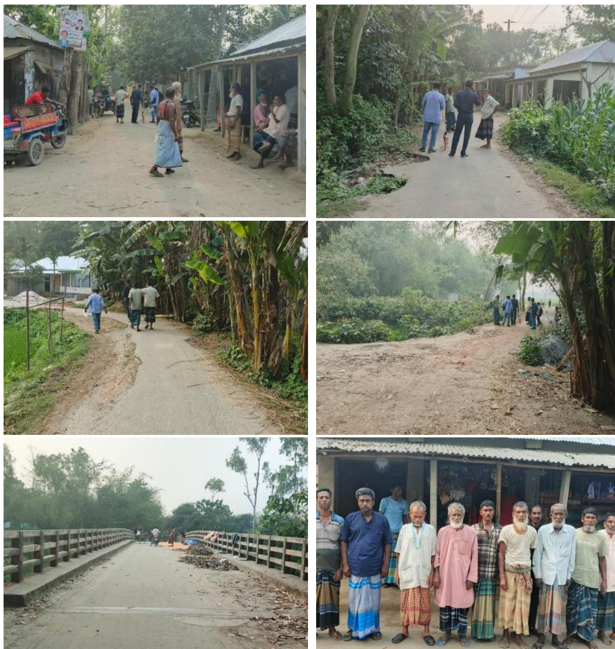
Existing Condition and the Surroundings of the Proposed Road
