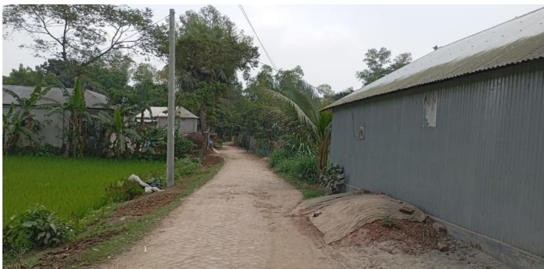
Starting Point of Chalapnra UZR-South Paikpara hat Road
