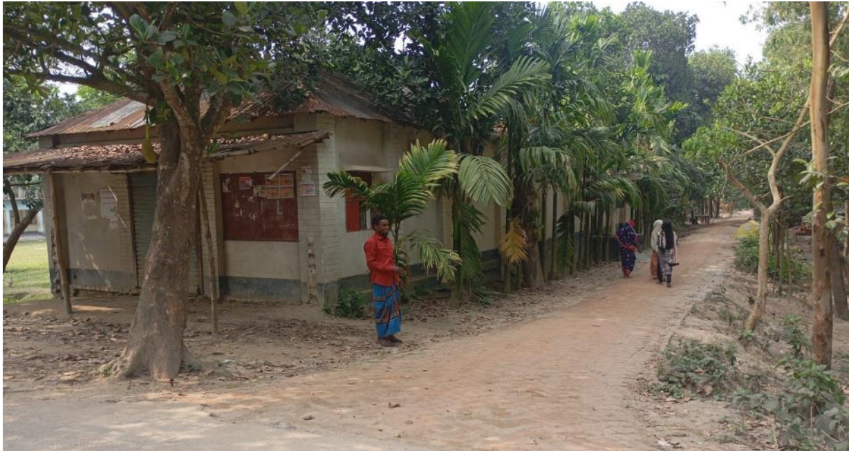
Starting Point of Jamirbaria-Uzgram Bazar Road
