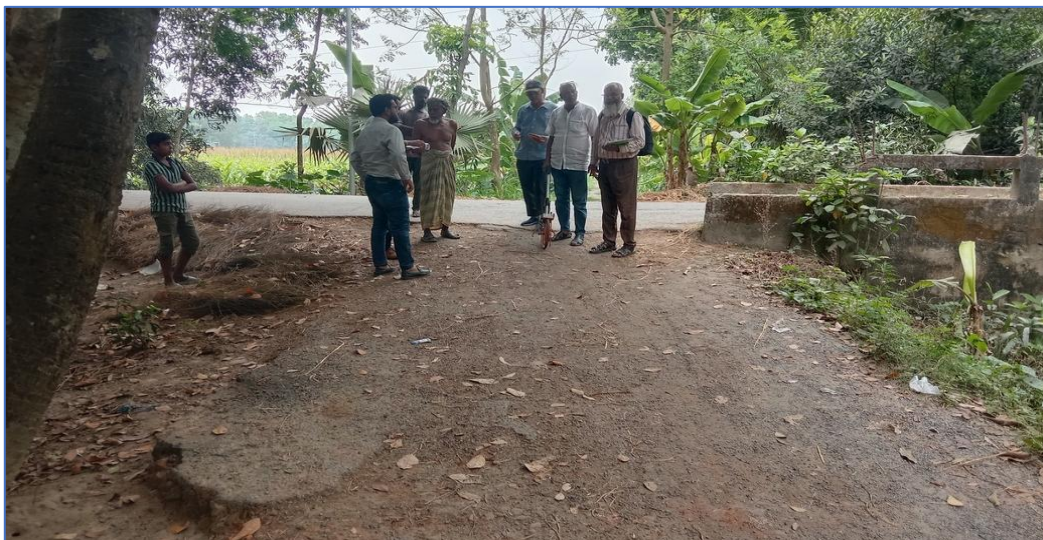
Starting Point of Bhuiyapara Care Road Bridge - Kathaldangi H/O Gopal Kazi
