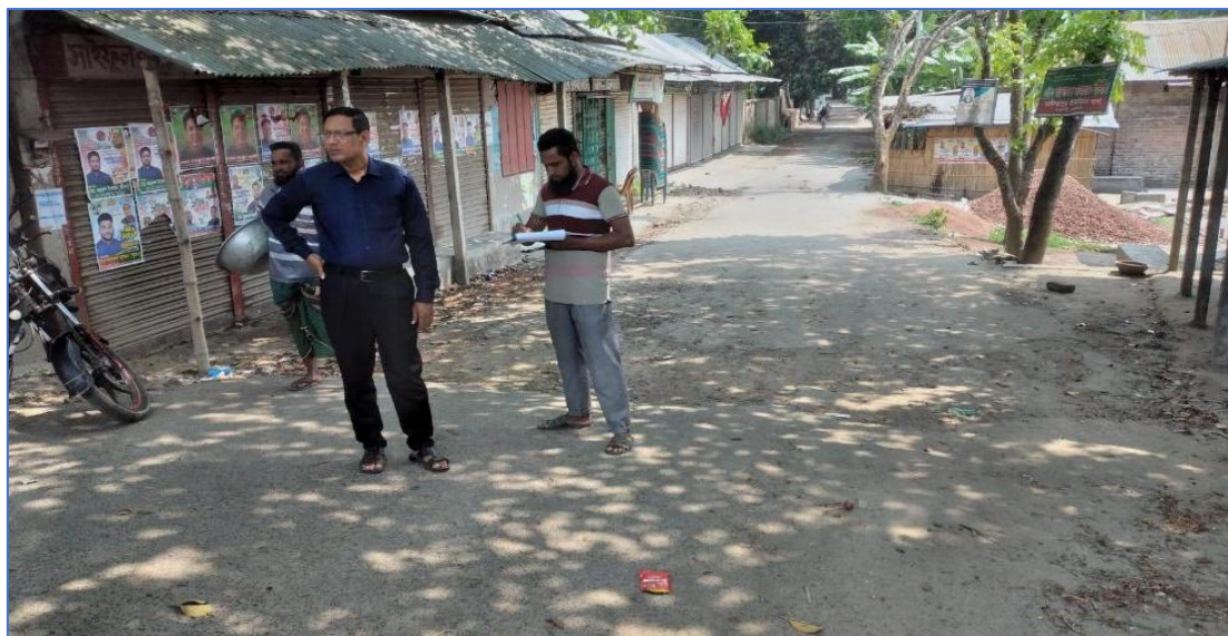
Starting Point of Kalikapur UP-Kalikapur Bazar Road
