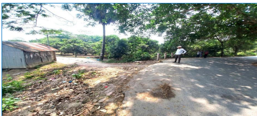
Starting Point Chanpathi-Kachabali Road
