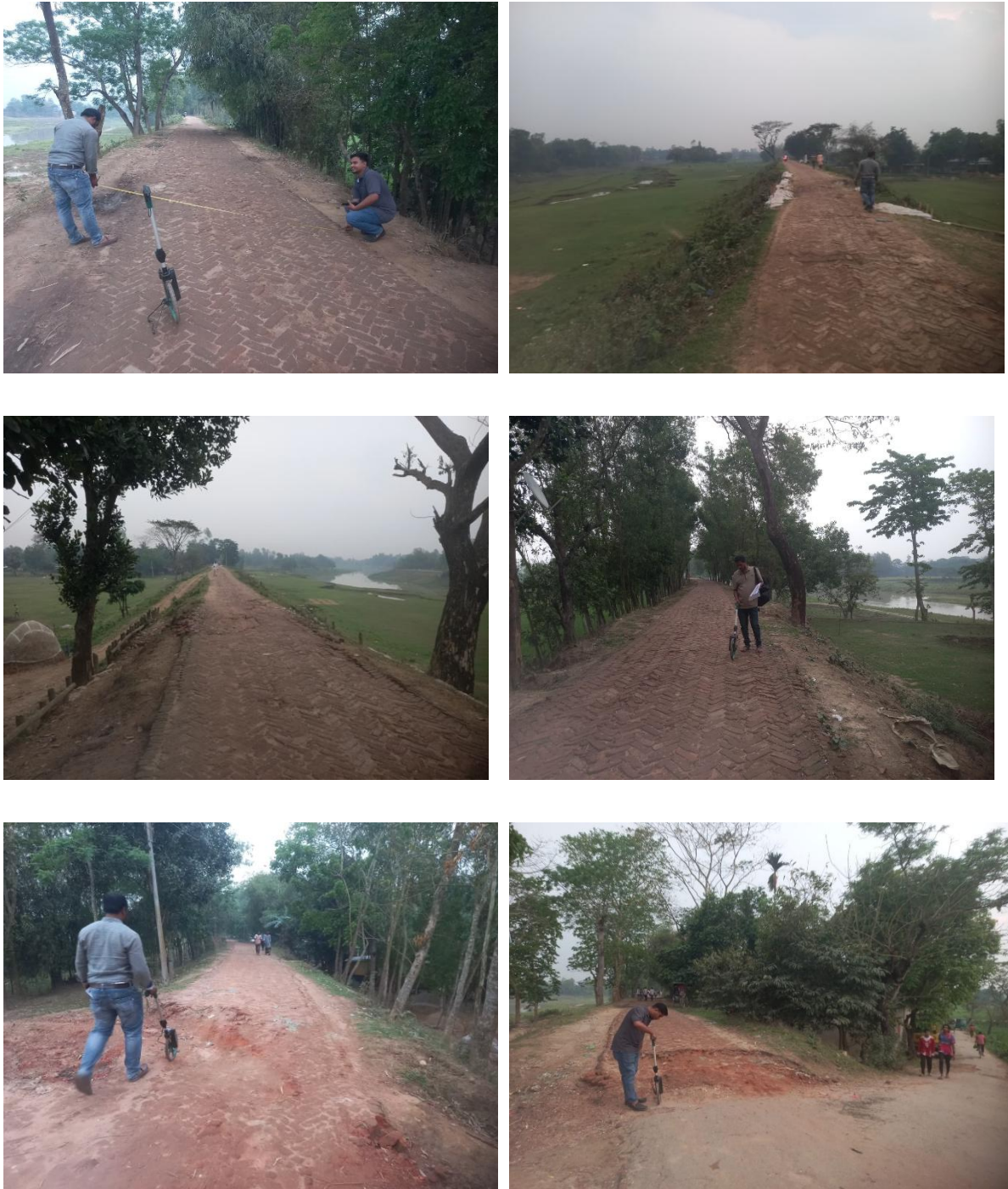
Figure: Existing Surroundings of the Sub-Project
