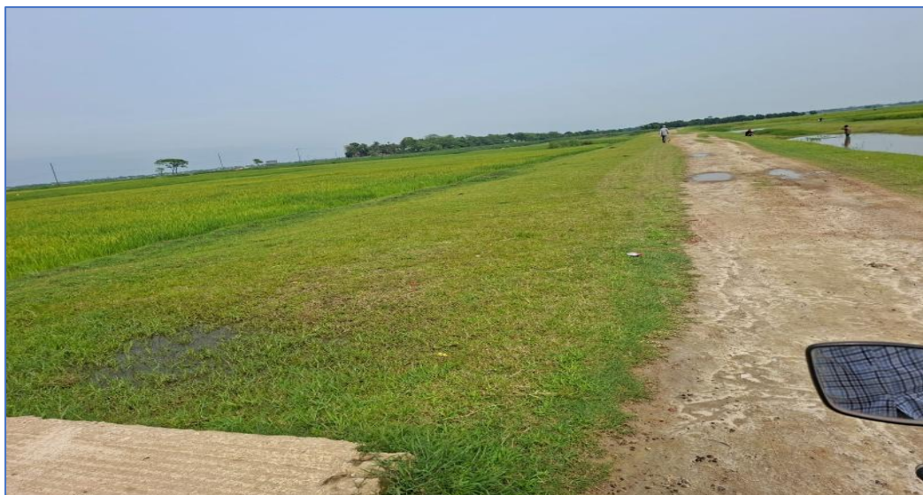
Starting Point of Sunamganj-Chhatak Road to Alampur via Shahpur-Monoharpur
