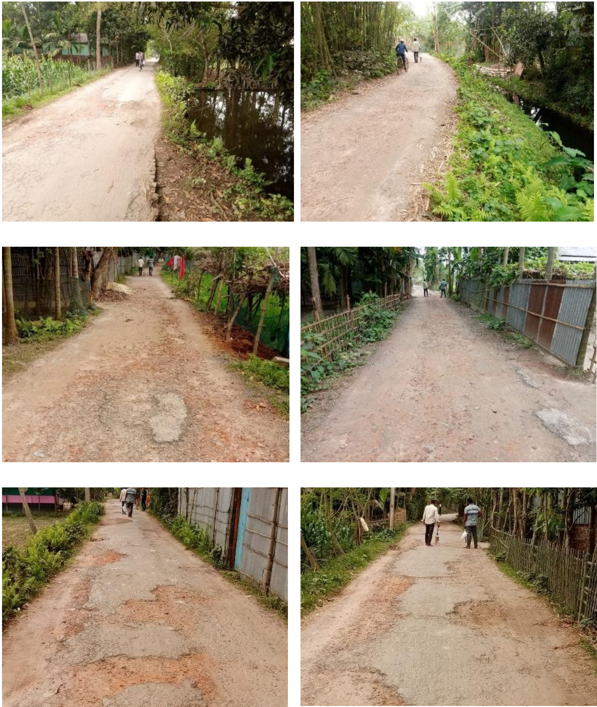
Figure: Existing Surroundings of the Sub-Project
