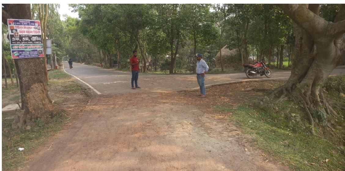
Starting Point of Shahjibazar-Sadurbazar road to Nurpur UP-Kesobpur Bazar Road
