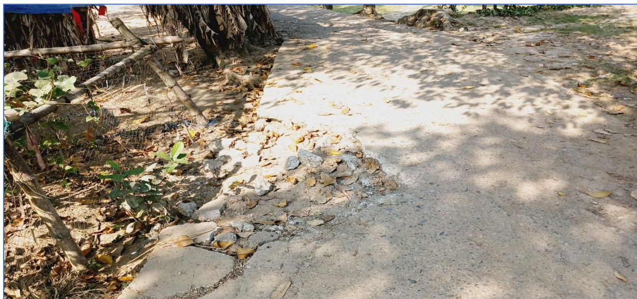
Starting Point of Baliura GCM (British Point)-Banglabazar GCM Road
