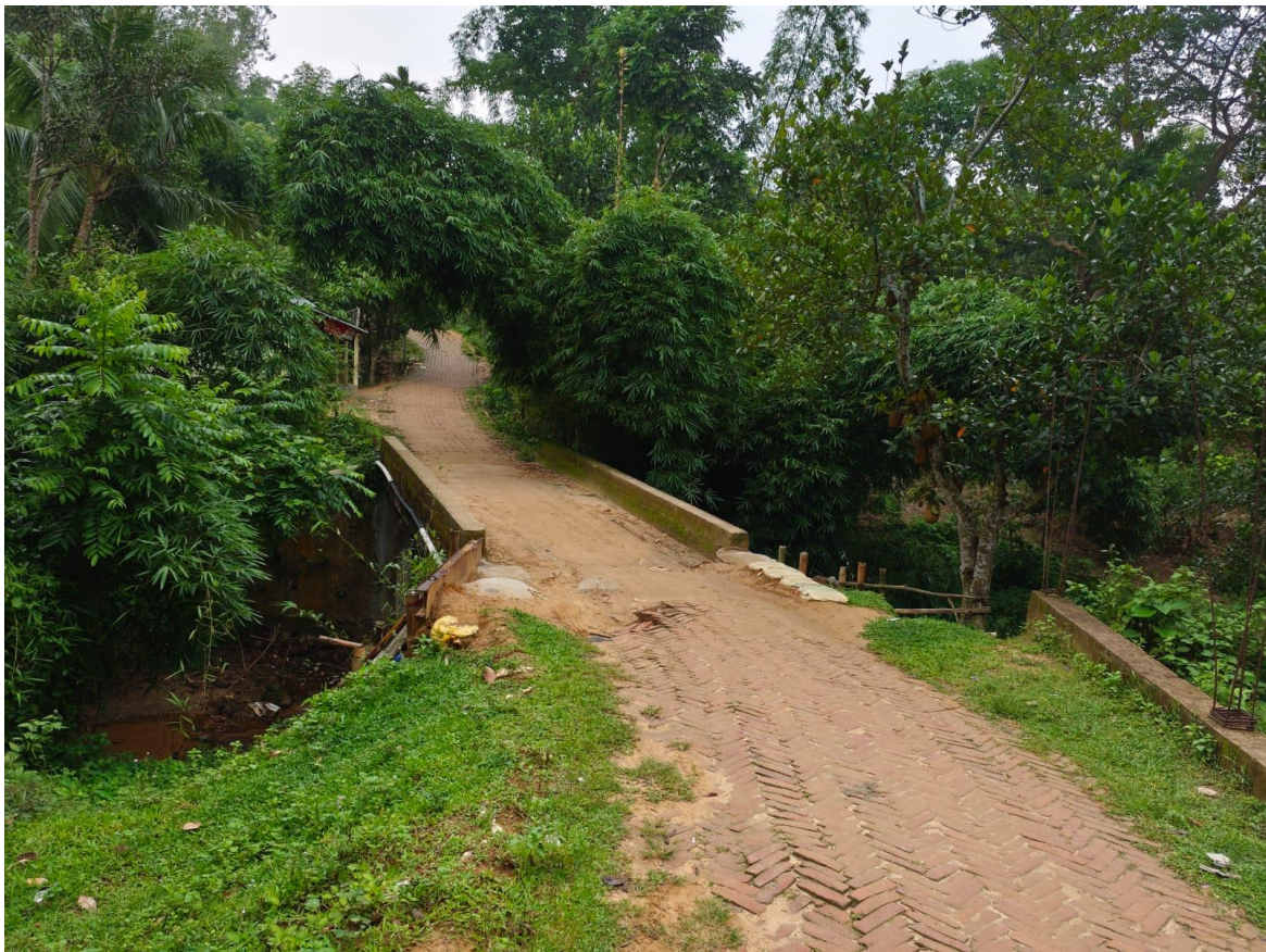
Photograph 2.2.3: Existing bridge condition of the Subproject Site
