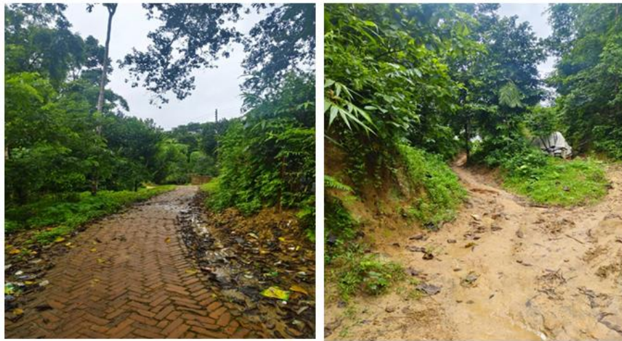
Photograph 2.2.1: Existing Road Condition of the Subproject Site
