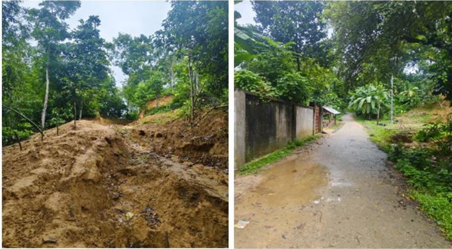
Photograph 2.2.2: Existing Road Condition of the Subproject Site
