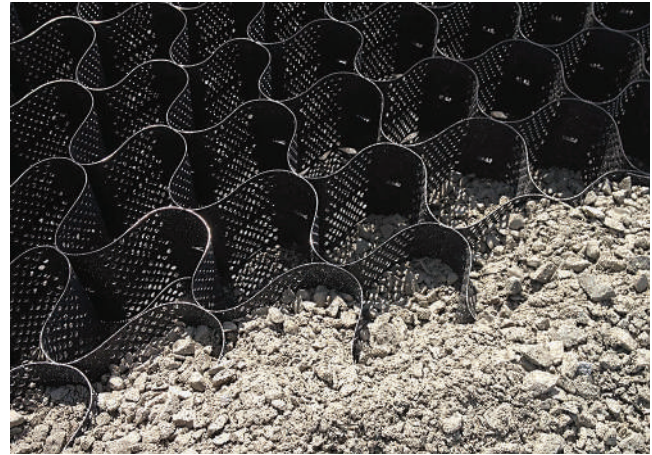
Figure 9. Geocells partly filled with aggregate
