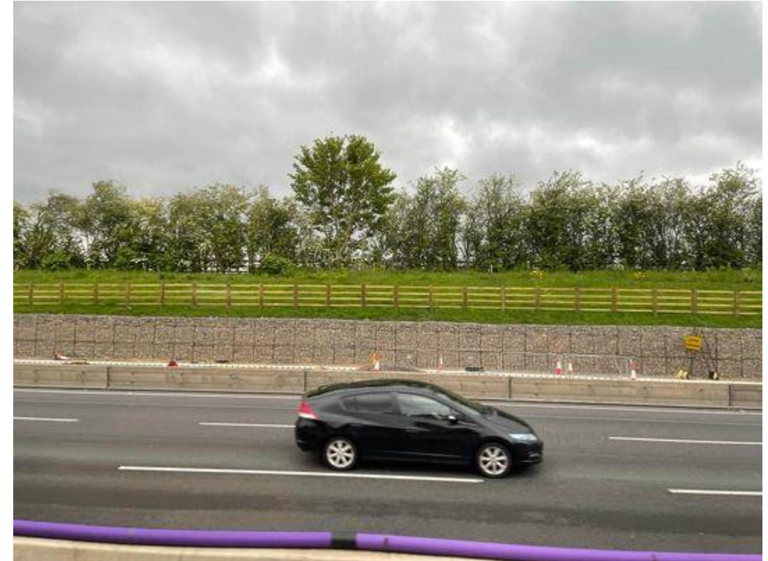
Figure 4 Retaining Structure Gabion Wall
