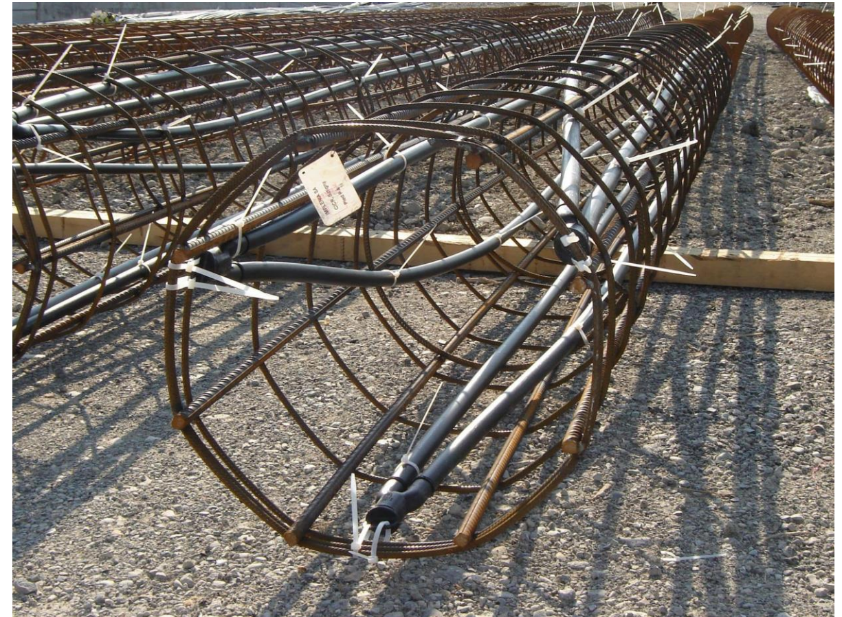
Figure 6.2 Energy pile
