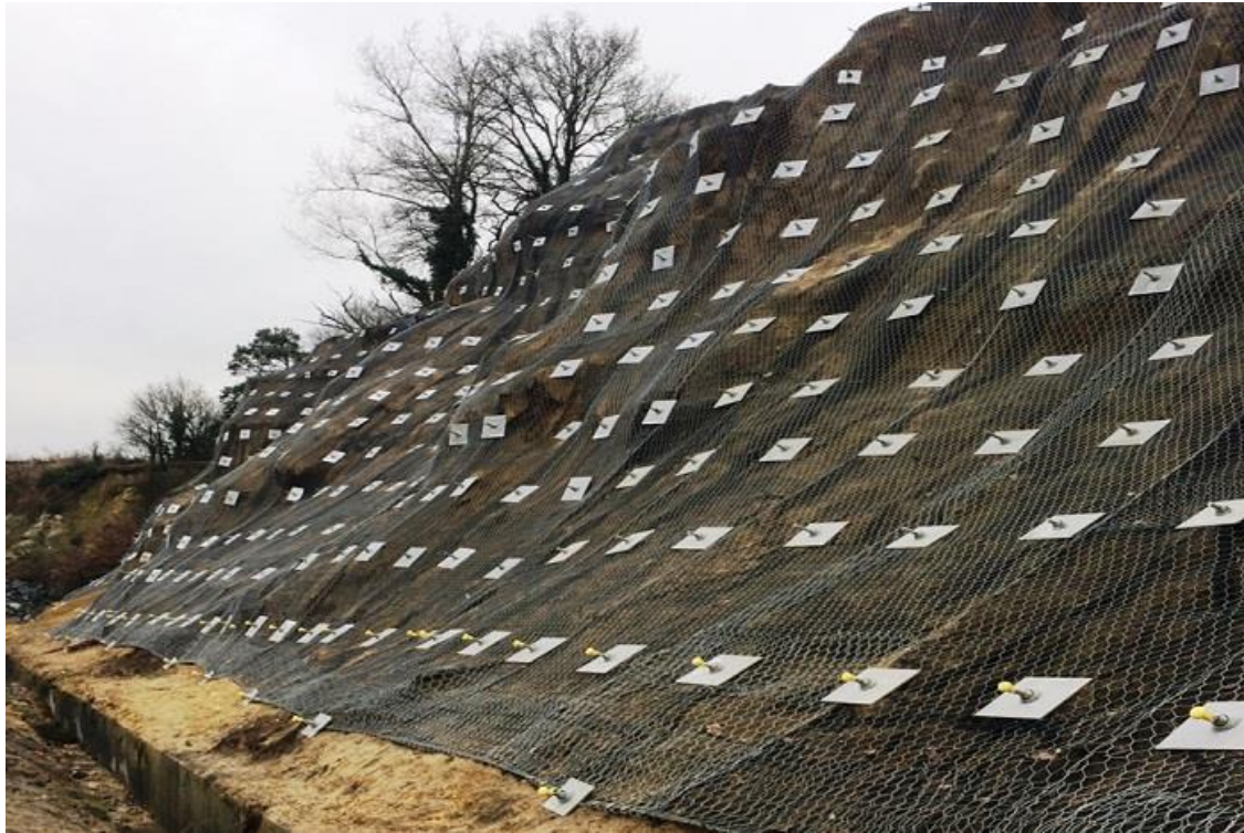
Figure 3 Retaining Structure Soil Nail
