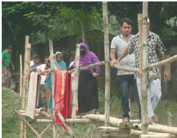
Figure 1.Existing Foot Bamboo Bridge Condition
