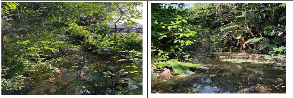
Photograph 2.2.2: Existing drain Condition of the Subproject Site
