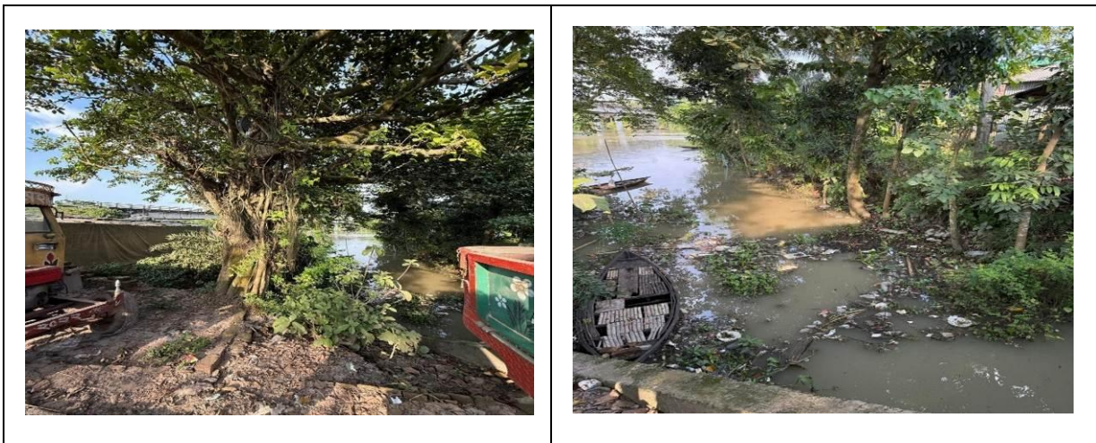
Photograph 2.2.3: Existing Road and drain Condition of the Subproject Site
