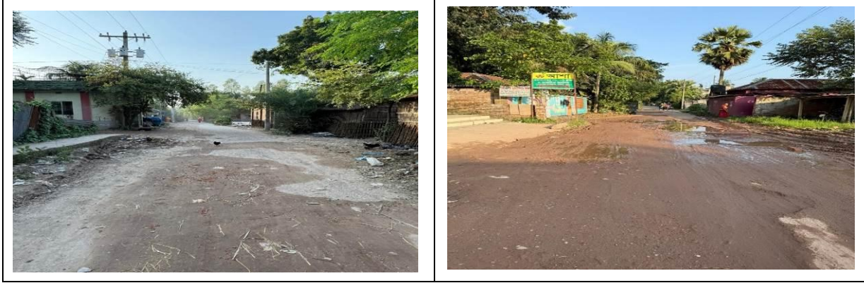
Photograph 2.2.1: Existing Road Condition of the Subproject Site
