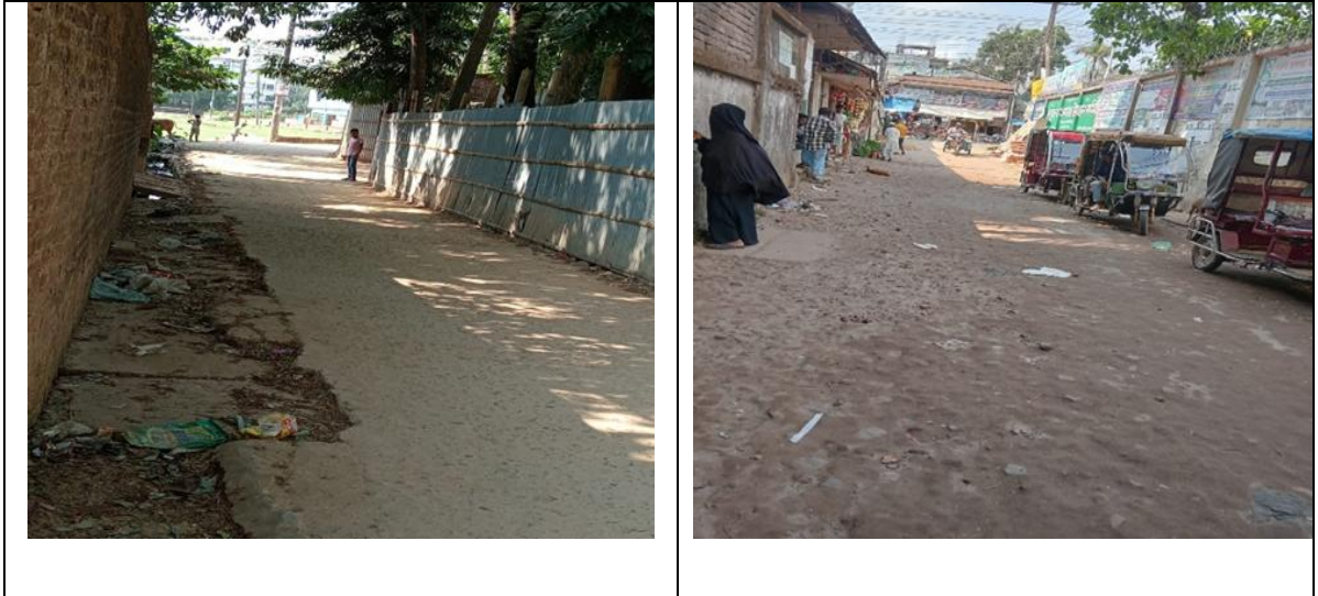
Photograph 2.2.1: Existing Road Condition of the Subproject Site
