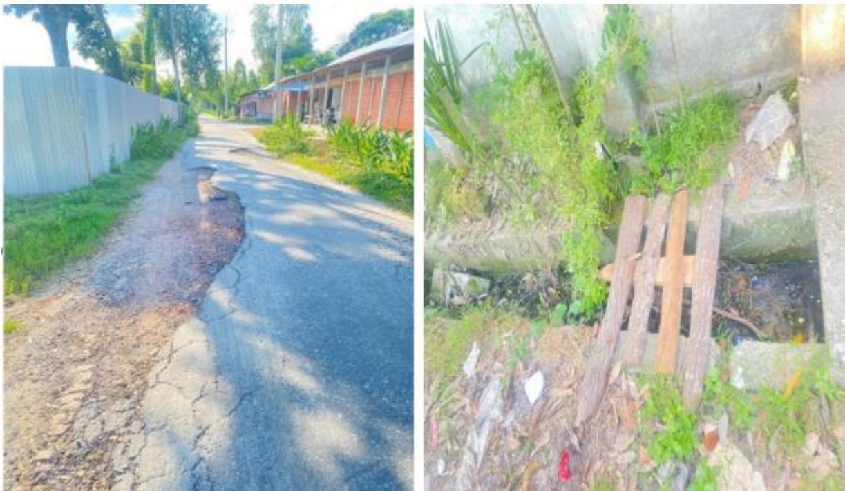
Photograph 2.2.2: Existing Road and Drain Condition of the Subproject Site
