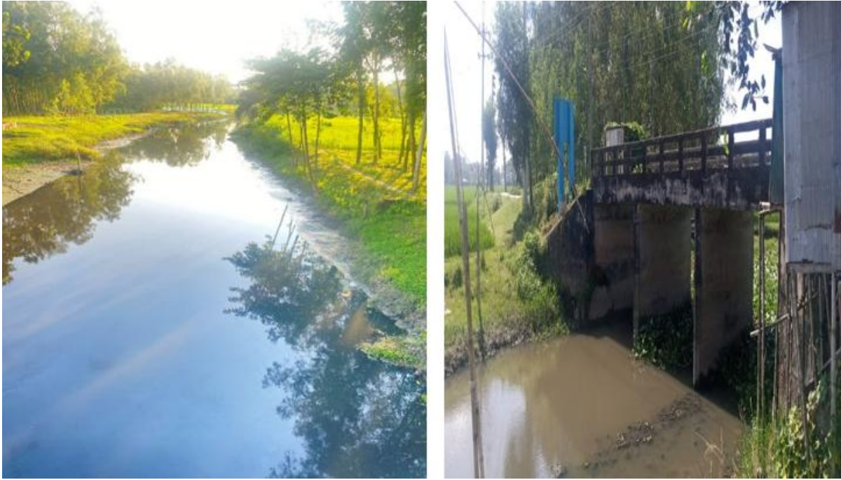
Photograph 2.2.3: Existing outfall of the Subproject Site
