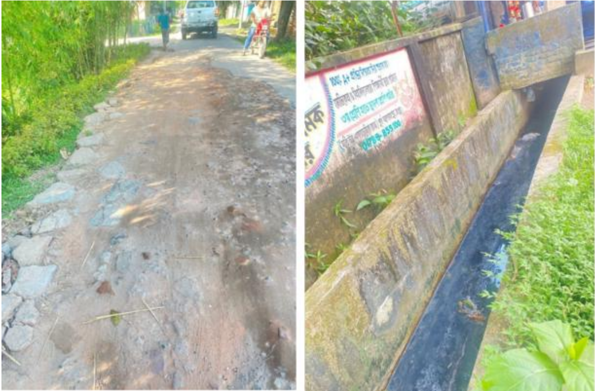
Photograph 2.2.1: Existing Road and Drain Condition of the Subproject Site
