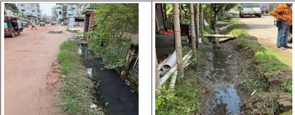
Photograph 2.2.2: Existing drain Condition of the Subproject Site
