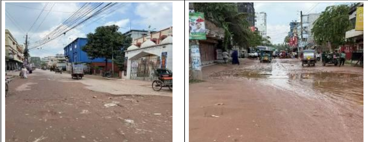
Photograph 2.2.1: Existing Road Condition of the Subproject Site
