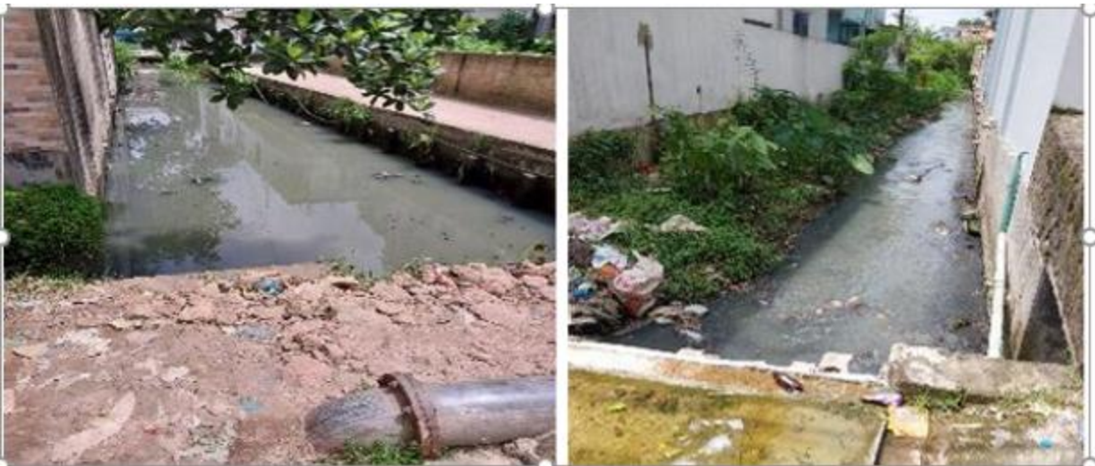
Photographs 2.2.2: Current Situation of the Outfall at Subproject Site
